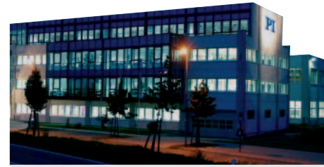
PI headquarters in Karlsruhe
